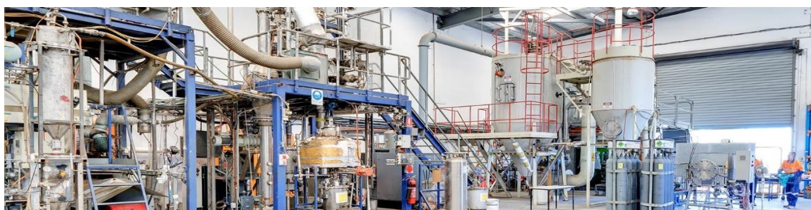
The VSPC cathode powder pilot plant and research facility.
