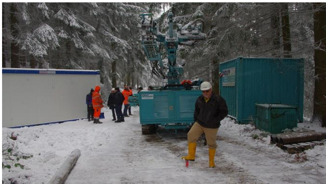
Figure 1. LIT managing director Adrian Griffin observes preparations for drilling at Sadisdorf.
