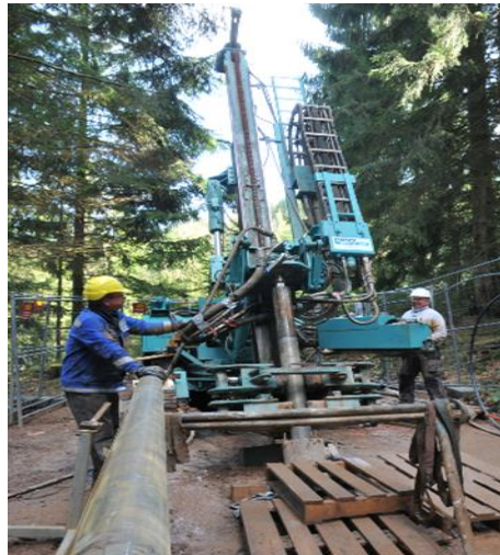
Figure 1 Drill rig at Sadisdorf
